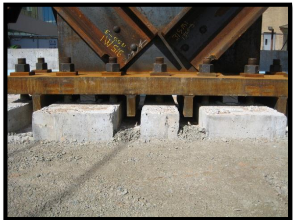
Figure 4 (Above): Picture of the braced frame connection to the foundation
