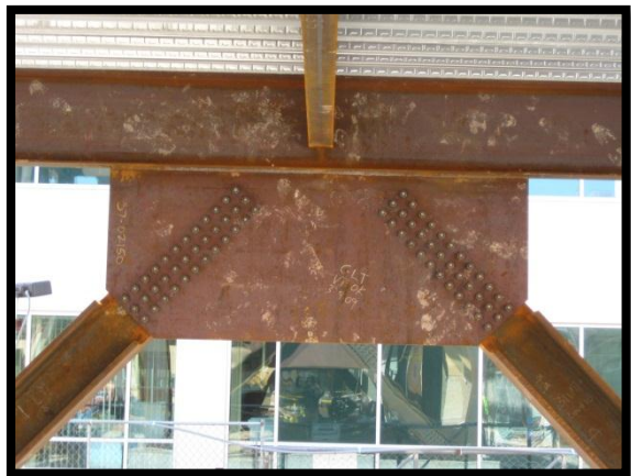
Figure 3 (Above): Close-up of gusset plate construction for the braced frame
