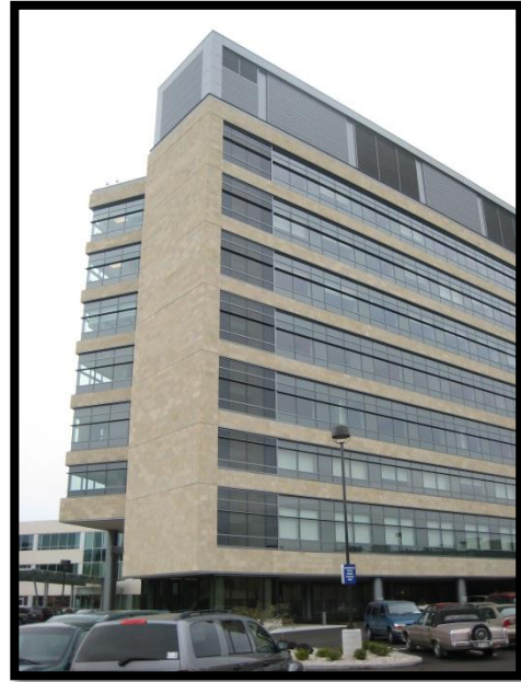
Picture 3: Bed Tower Addition
